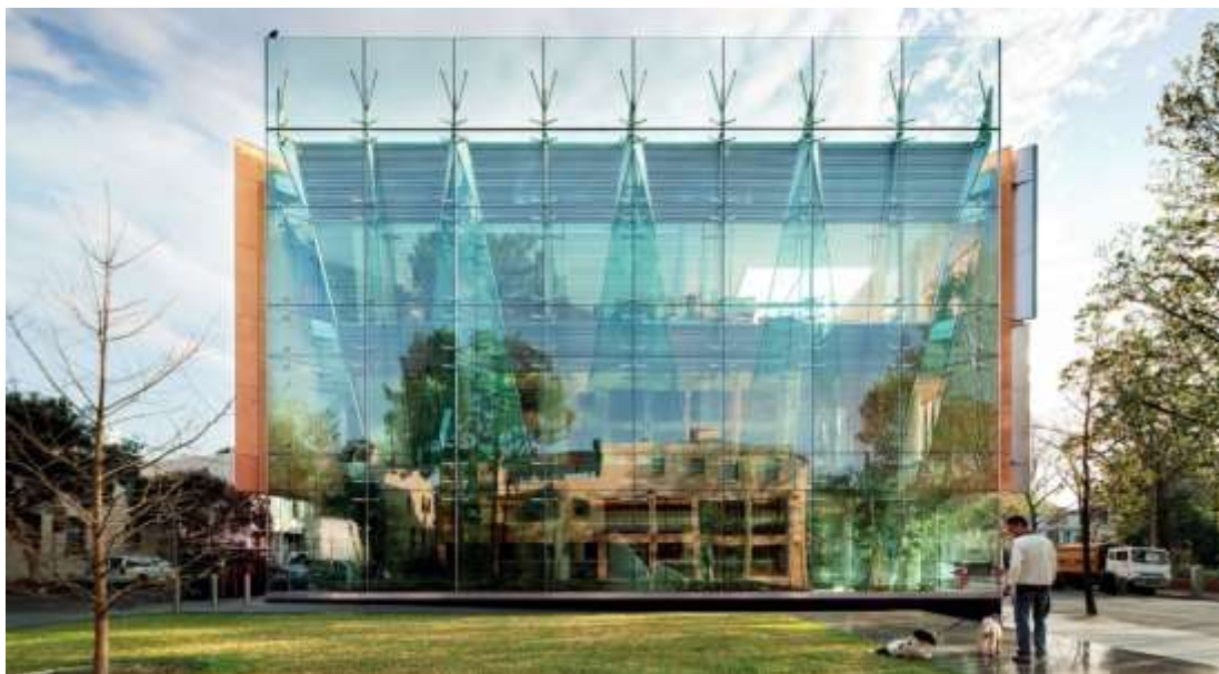
Transparency and connection were the underlying principles in the design of the Surry Hills Library by fjmt. Photo – Courtesy of Surry Hills Library.
